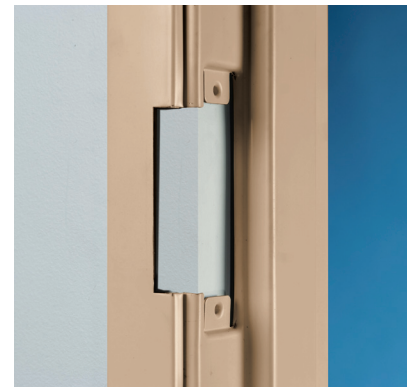
Electric Strike Prep with Casing Notch
