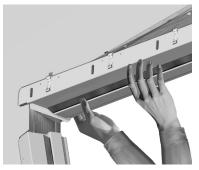
Sleeve the hinge jamb over the wall. Bring the header down tight, interlocking the stop in the alignment tab. Try to place the hinge jamb close to the stud to
